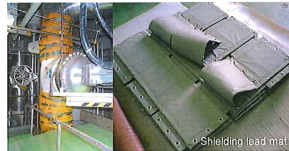
Laminated thin-plate lead mat (pipe shield) Lead wool
